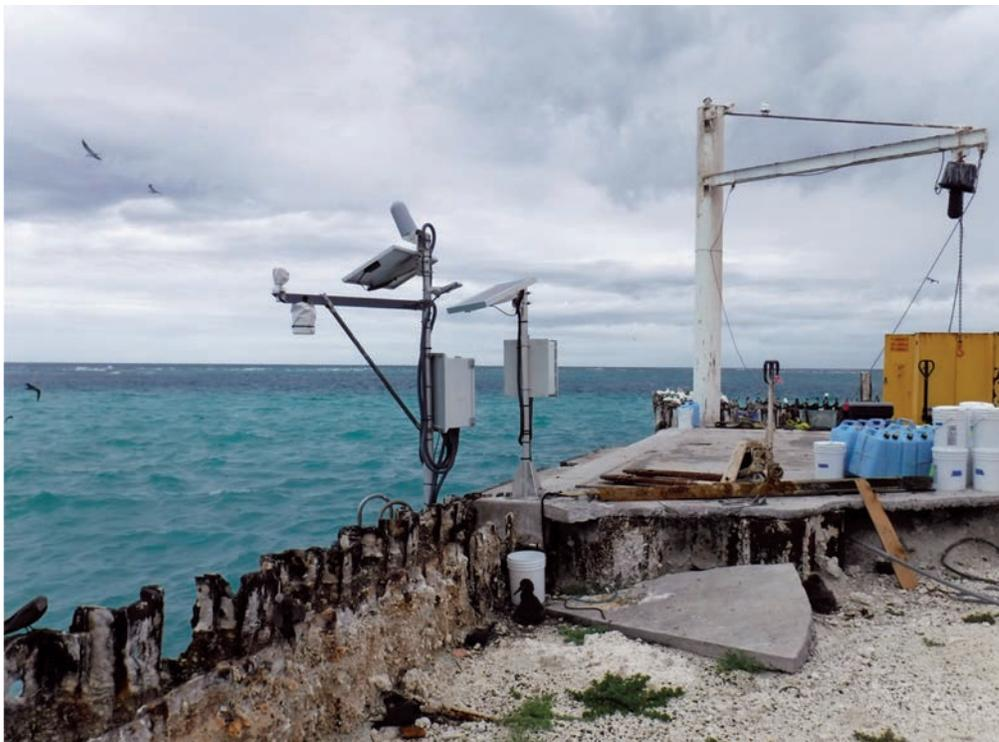
*Figure 1. Rebuilt tide gauge installation on Tern Island in French Frigate Shoals, which was previously destroyed by Hurricane Walaka. Portions of the pier destroyed by the hurricane are visible in the foreground; the gauge is installed on a remaining stable portion of the pier.*
