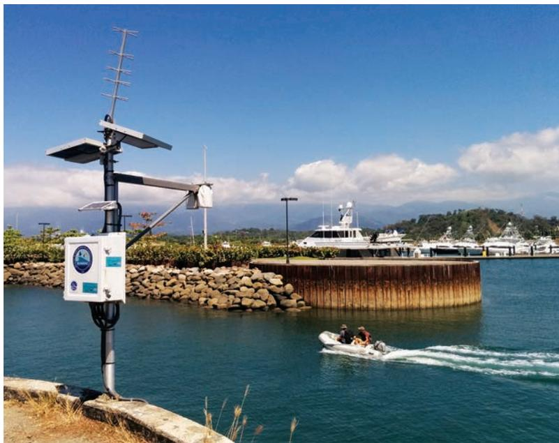
*Figure 1. UHSLC tsunami water level station at Quepos, Costa Rica.*
